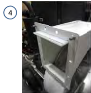
Liner at outlet position when fully inserted
