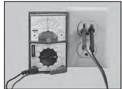
(F) Check power source voltage is 120v - if not 120v, move to another circuit
