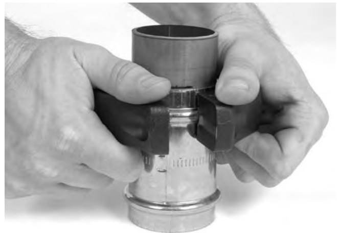
Figure 8 – Installing Press Ring Onto Fitting
